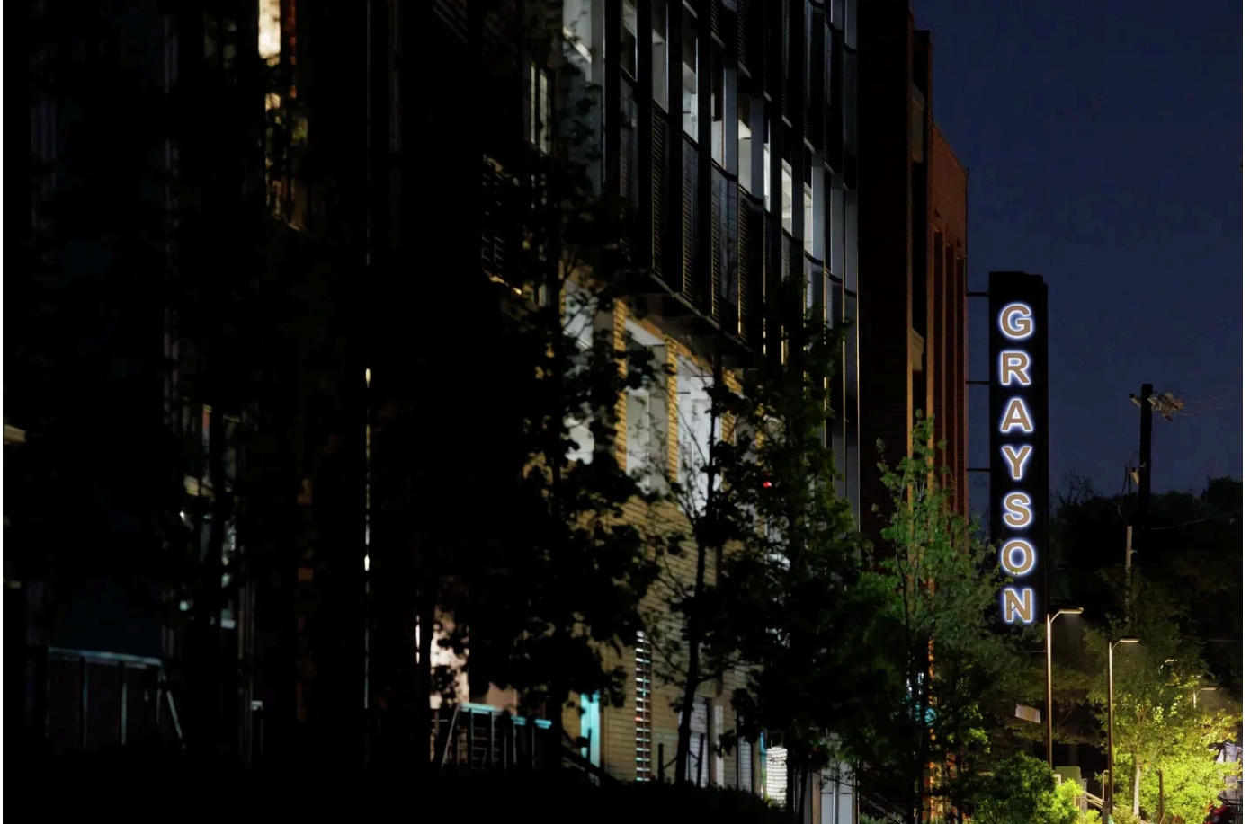
The Residences at Grayson Heights is a new apartment complex in San Antonio’s Government Hill neighborhood. A steady stream of water is flowing from the complex’s parking garage, pooling on nearby roads and drawing complaints from nearby residents. Sam Owens/San Antonio Express-News
