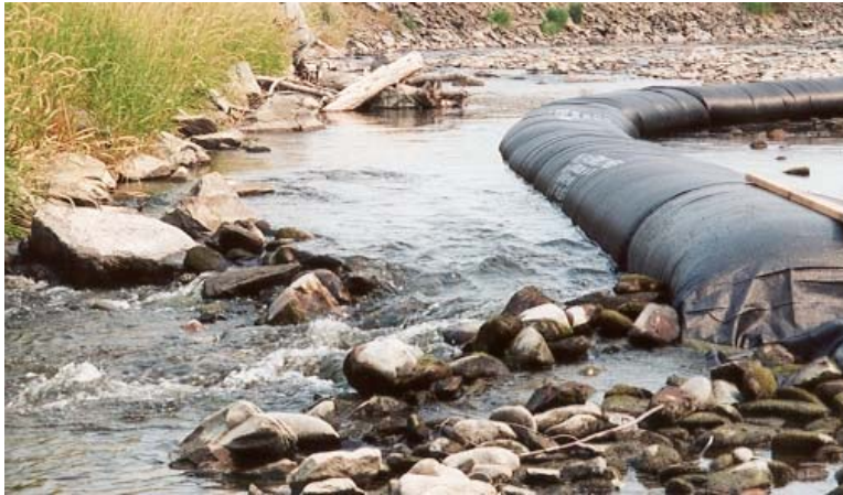
Figure 42. Aqua Dam inflatable cofferdams
