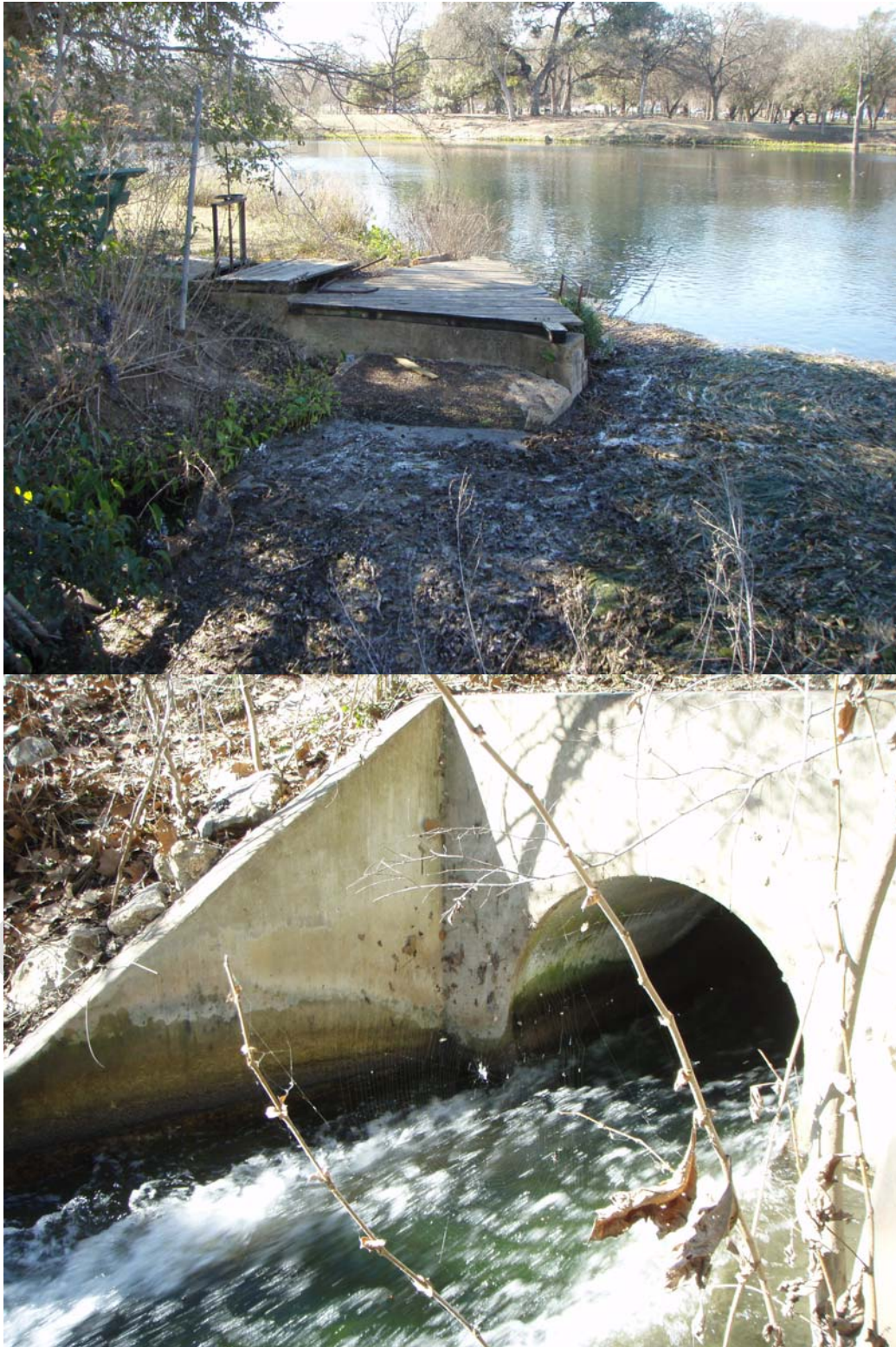
Figure 2. New 48-inch culvert from Landa Lake to the Old Channel
