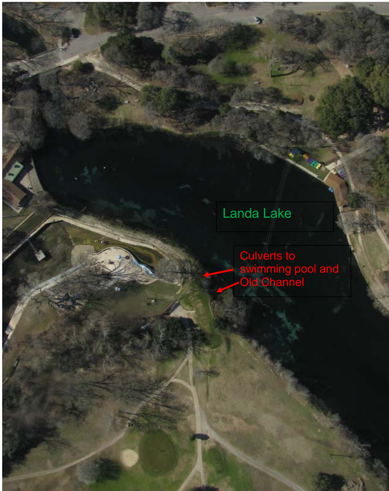
Figure 22. Landa Lake and culverts going to swimming pool and Old Channel
