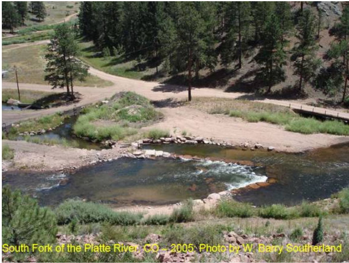
Figure 28. Rock cross vane weir, South Fork Platte River, Colorado
