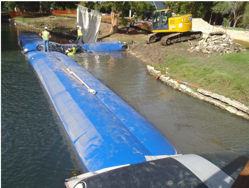
Figure 6: Landa Lake walls construction project – upstream view towards Spring run 2.
