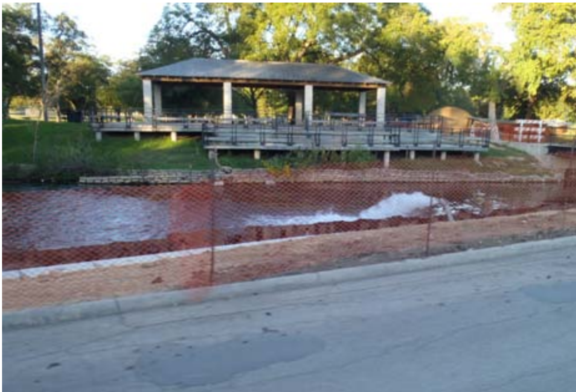
Figure 8: Walls construction project in the New Channel.
