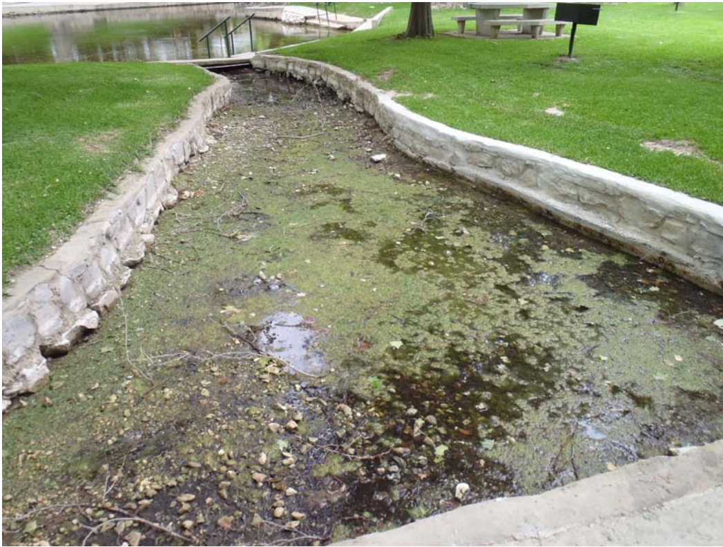
Figure 6: Stagnant conditions in southern channel of Spring Run 6 on Spring Island
