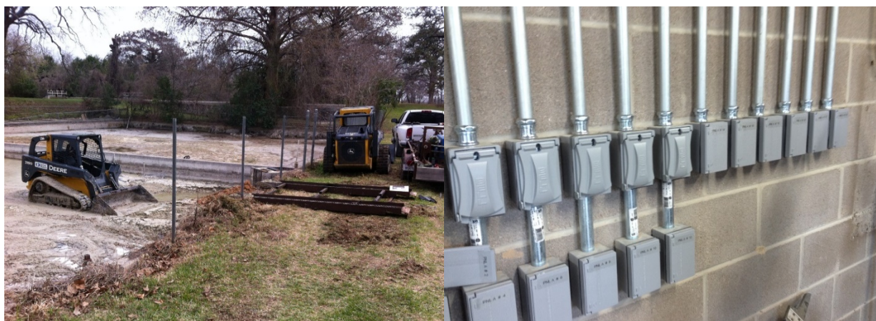
Figure 3.1-2. Draining and dredging of the outdoor ponds (left) and installation of new electrical system (right)
