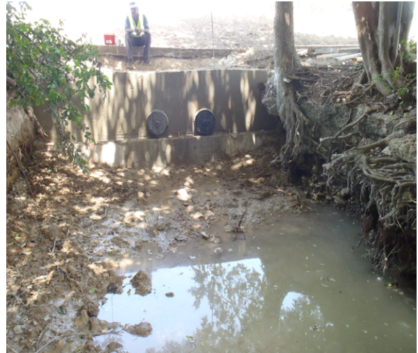
Figure 3.2-4. Two 24-inch culverts outlets to the Old Channel of the Comal River (following capping)
