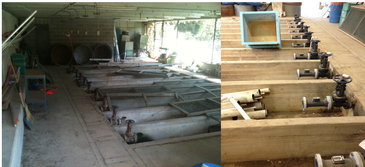
Figure 3.1-1. Replacement of aged troughs (left) with new valves and gauges (right)
