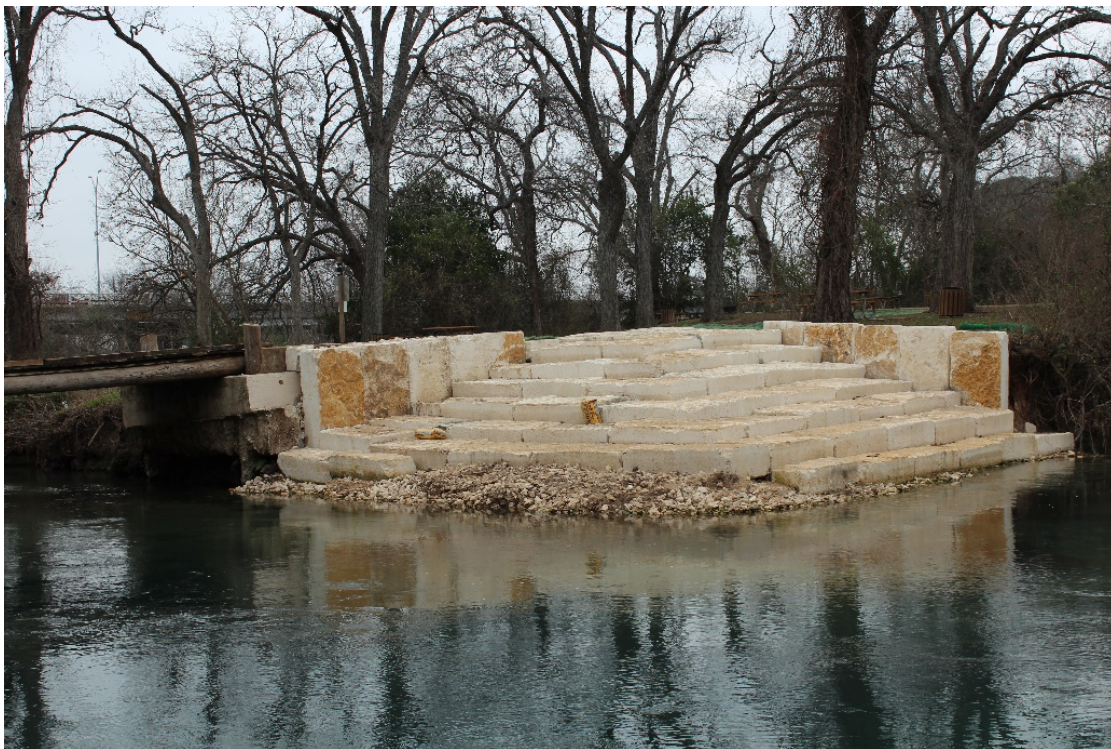
Figure 3.3-17. Upper access point at Ramon Lucio Park prior to modifications due to undermined lower level of rock.
