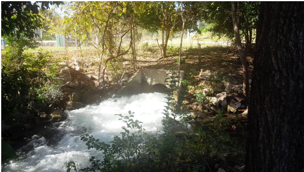
Figure 3.2-8. 48-inch culvert flowing from Landa Lake into Old Channel
