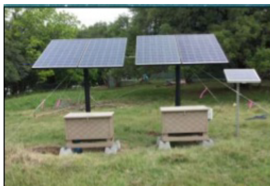
Figure 3.2-15. Solar panels that power the aerators
