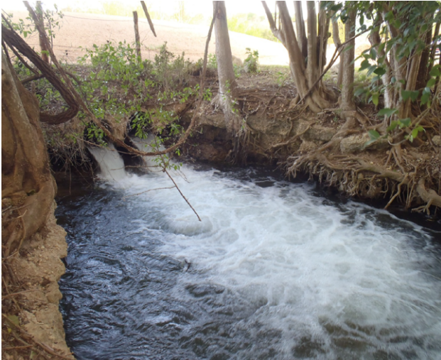
Figure 3.2-3. Two 24-inch culvert outlets to the Old Channel of the Comal River (prior to capping)
