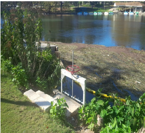
Figure 3.2-5. Flow Control Gate Structure (A)
