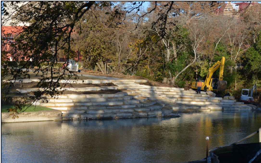
Figure 3.3-13. Natural rock was used to build bank stabilization/access points. This is the first of seven access points; called Dog Beach and located across from City Park
