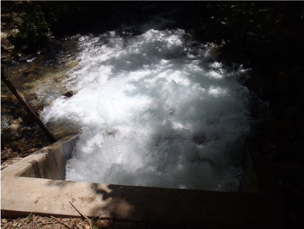
Figure 3.2-7. New culvert outlet into the Old Channel of the Comal River
