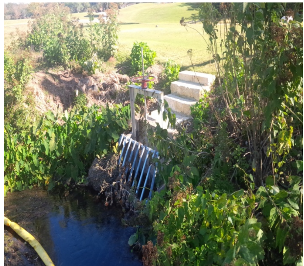
Figure 3.2-6. Flow Control Gate Structure (B)
