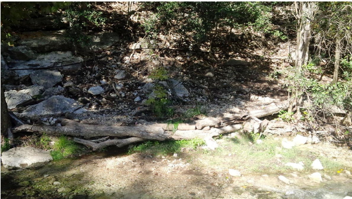
Figure 3.2-43. Structure built to capture erosion before entering Spring Run 3
