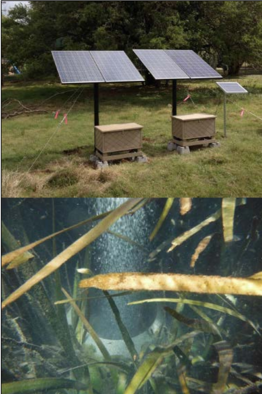
Figure 3-9. Aerator and water quality study equipment (top – aerator systems, telemetry unit, and their solar panels; bottom – submerged view of aerator diffusers in operation) (SWCA 2013a).
