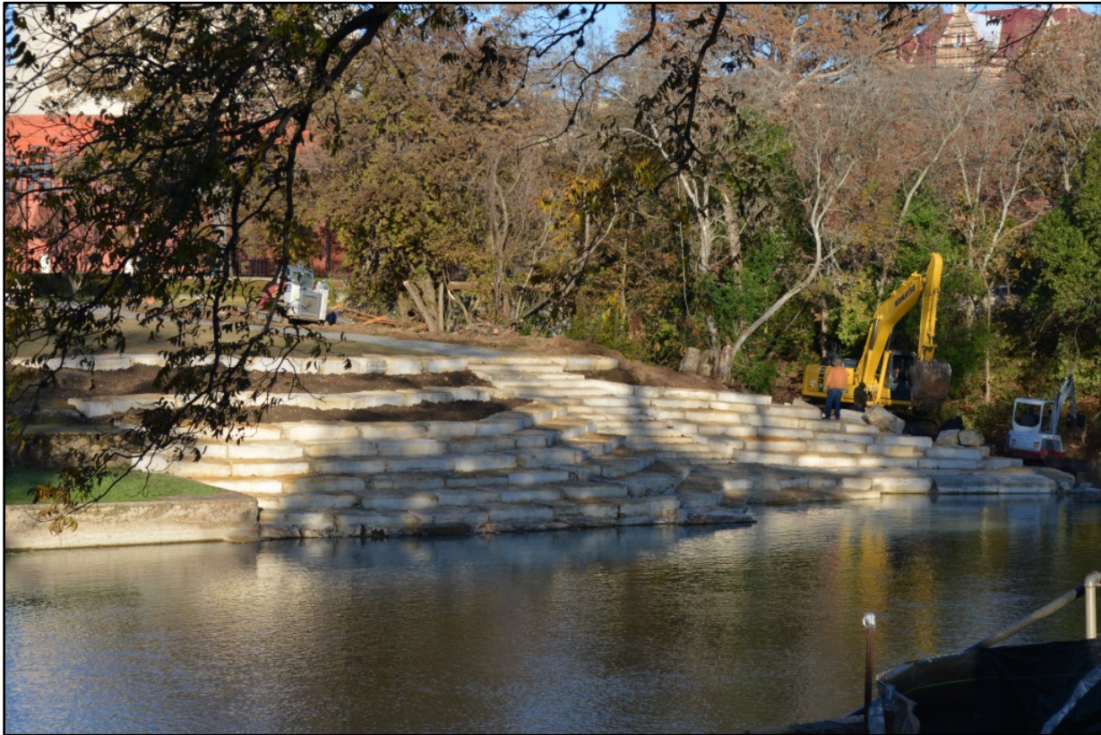
Figure 3-35. Natural rock was used to build bank stabilization/access points.
