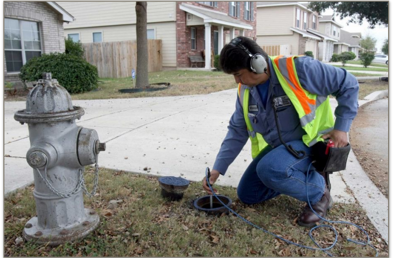
SAWS technician listens for leaks on water mains.
