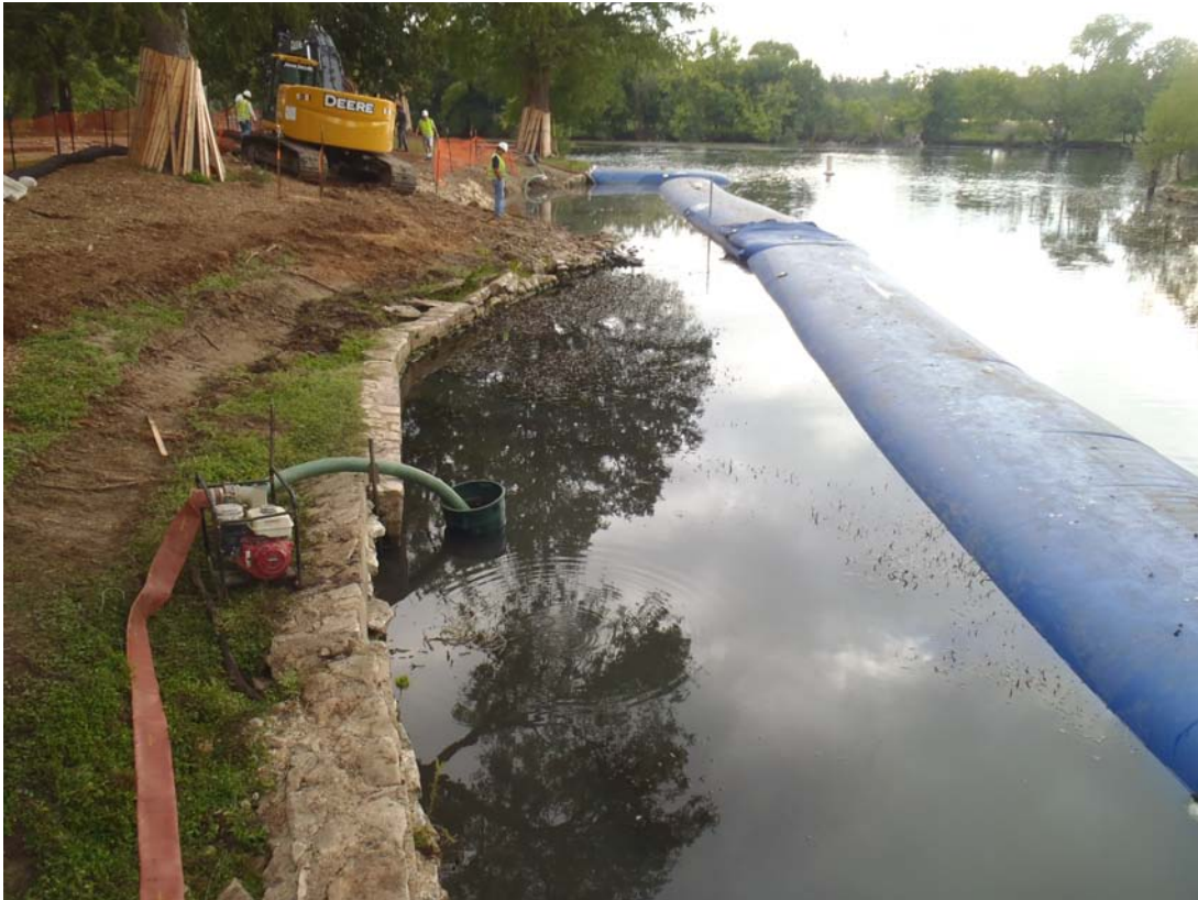
Figure 6: Landa Lake walls construction project - downstream view towards the lake.
