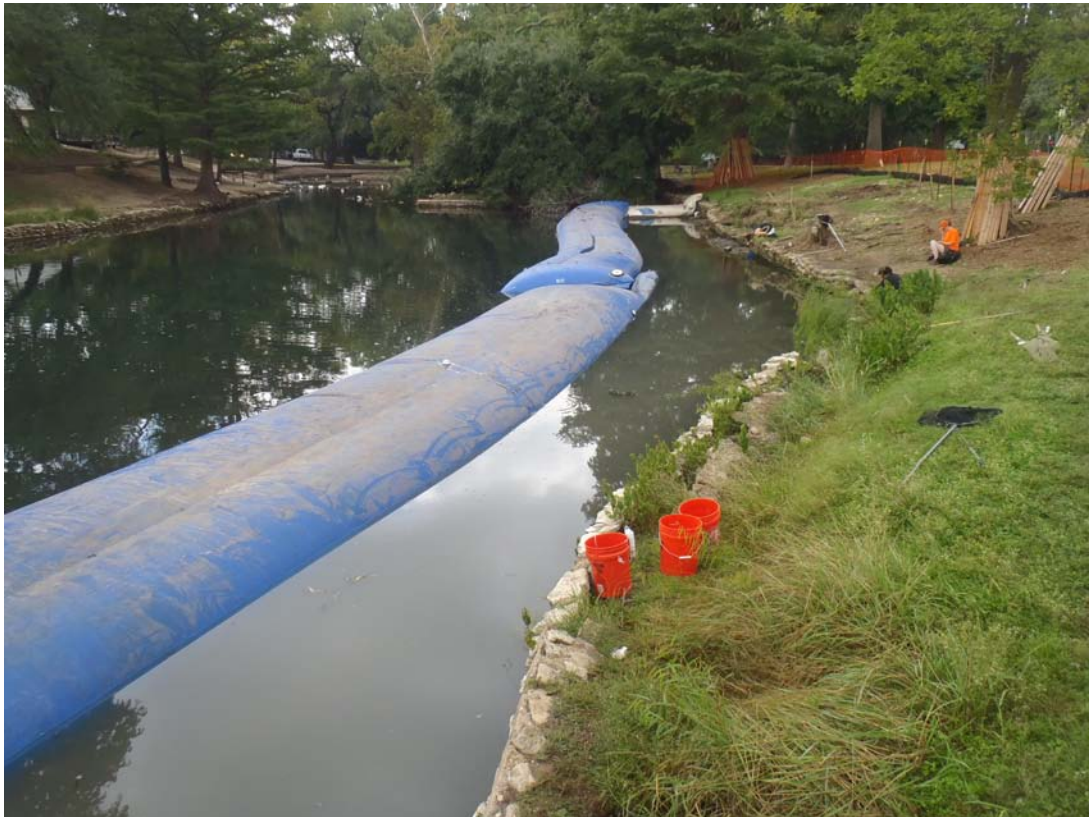
Figure 7: Landa Lake walls construction project – upstream view towards Spring run 2.
