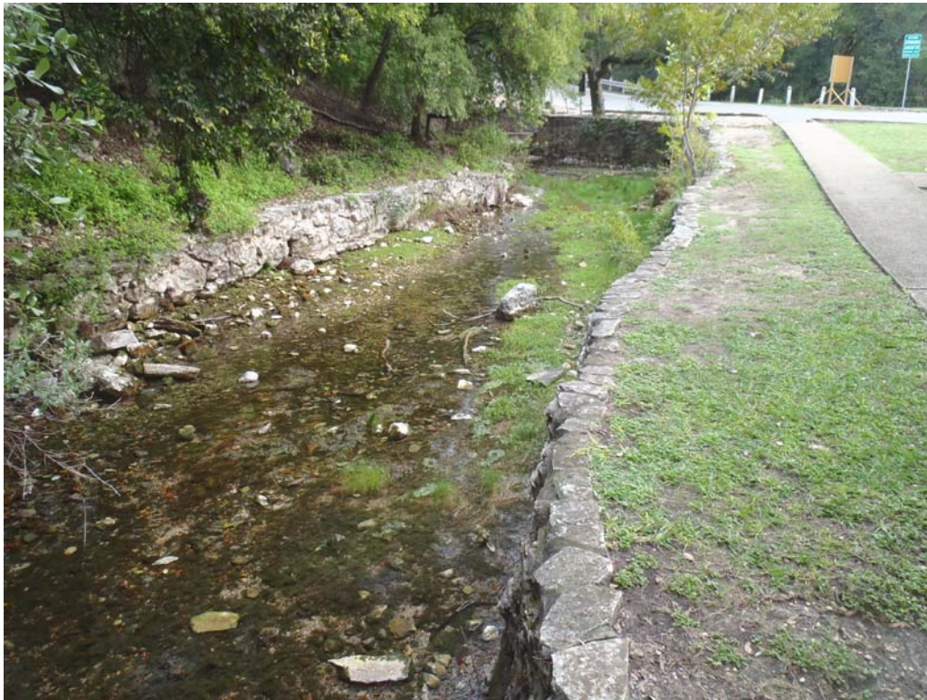
Figure 3: Looking upstream toward Spring run 1 main orifice. Continuous surface flow on river right (left side of photo).
