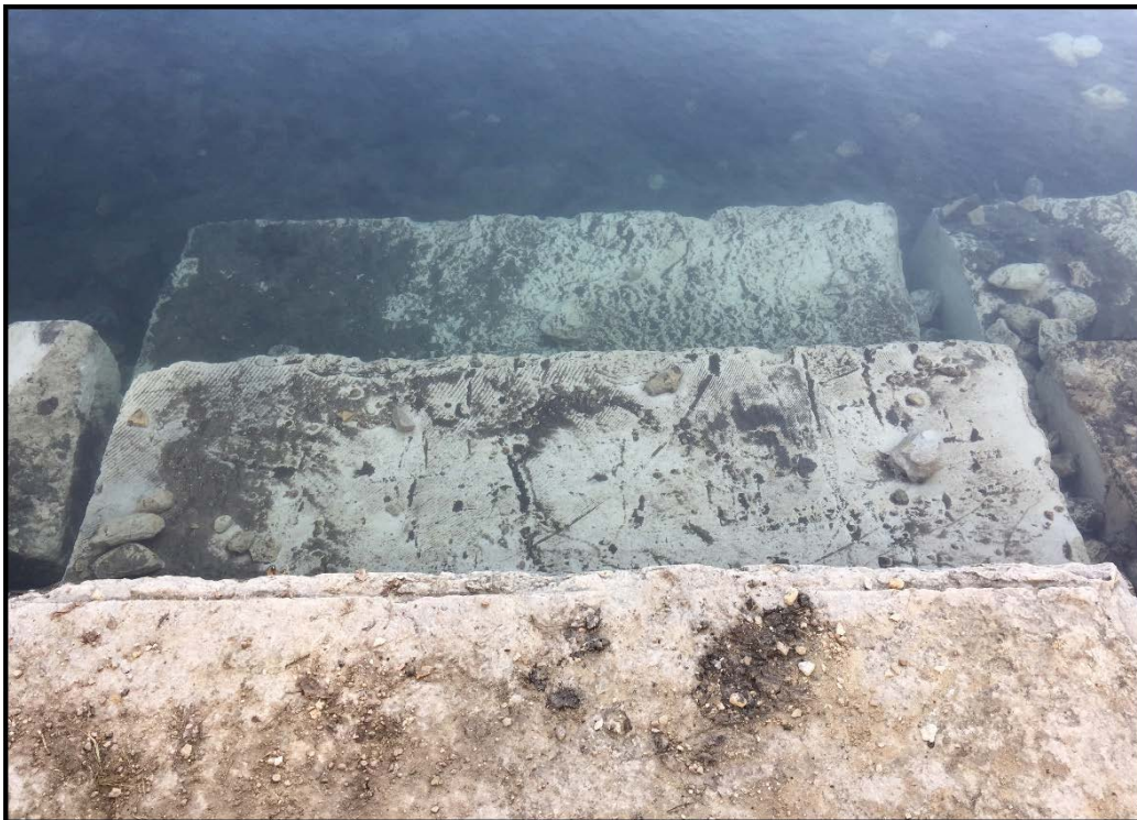
Figure 3.3-14. Portion of the installed anchor rocks at Hopkins Railroad Bridge access point.
