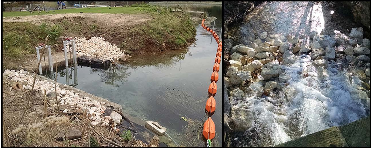
Figure 3.2-1. Back-up flow control gates and booms (left photo), and flow issuing into Old Channel from Landa Lake via new back-up flow controls gates and 14" culverts (right photo).
