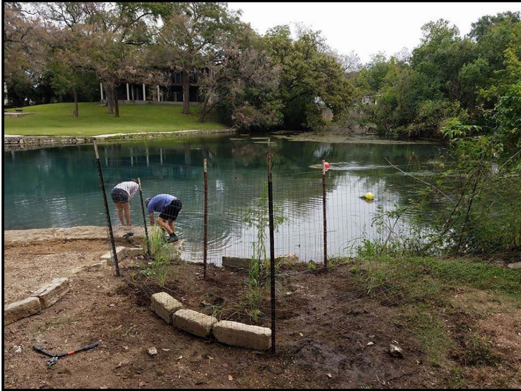
Figure 3.3-42. Bank erosion control through native plantings.
