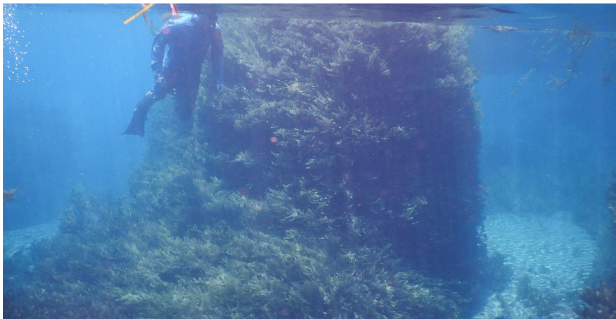
Appendix A4. Vegetation buildup on the anchor cables and outside end of boom 2.
