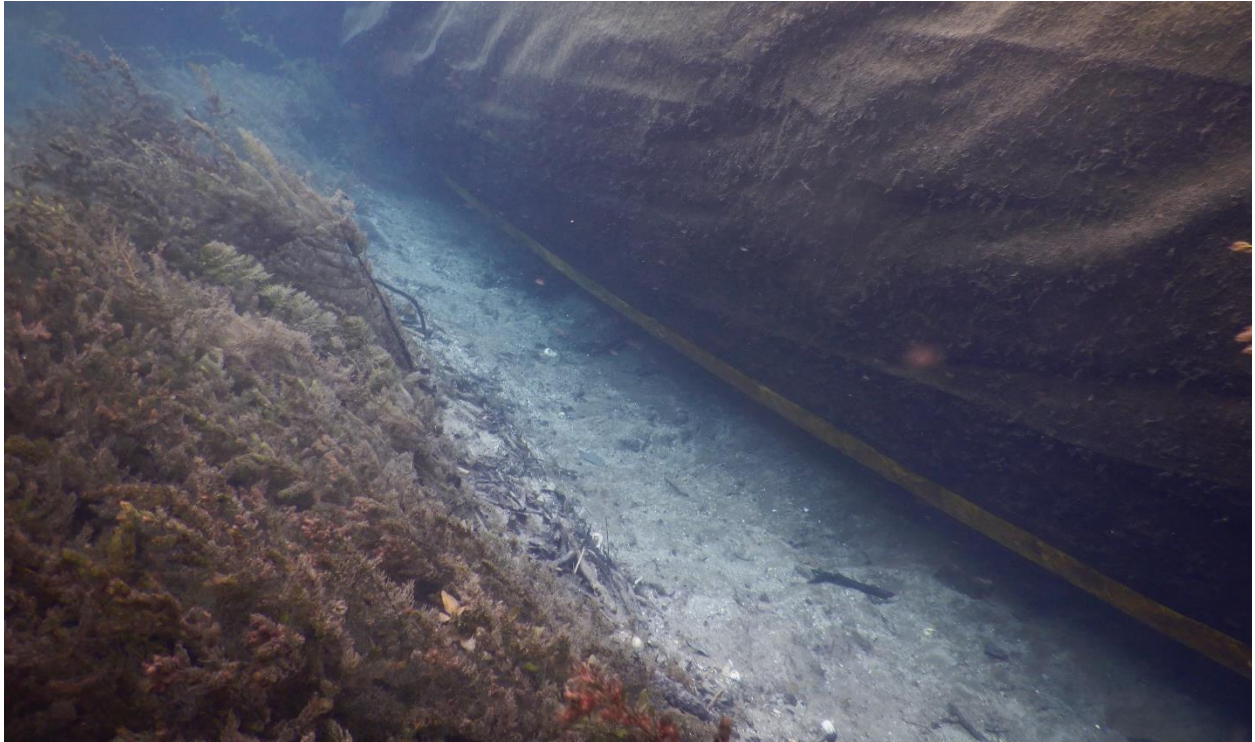
Appendix A11. Custom boom 3 before removal showing the buildup of sediment behind the boom due to harvester activity pushing excess water under the boom during removal efforts.
