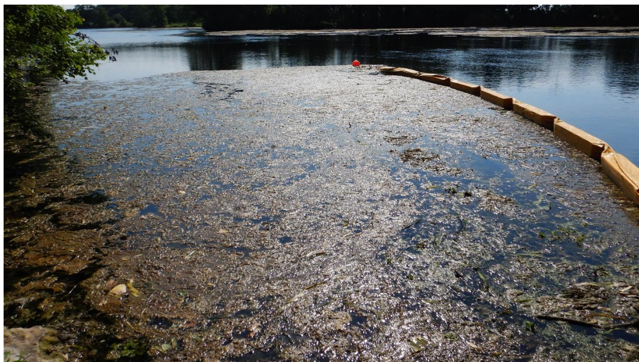
Appendix A10. Temporary boom 3 setup near full capacity showing what it looks like before harvester collection.
