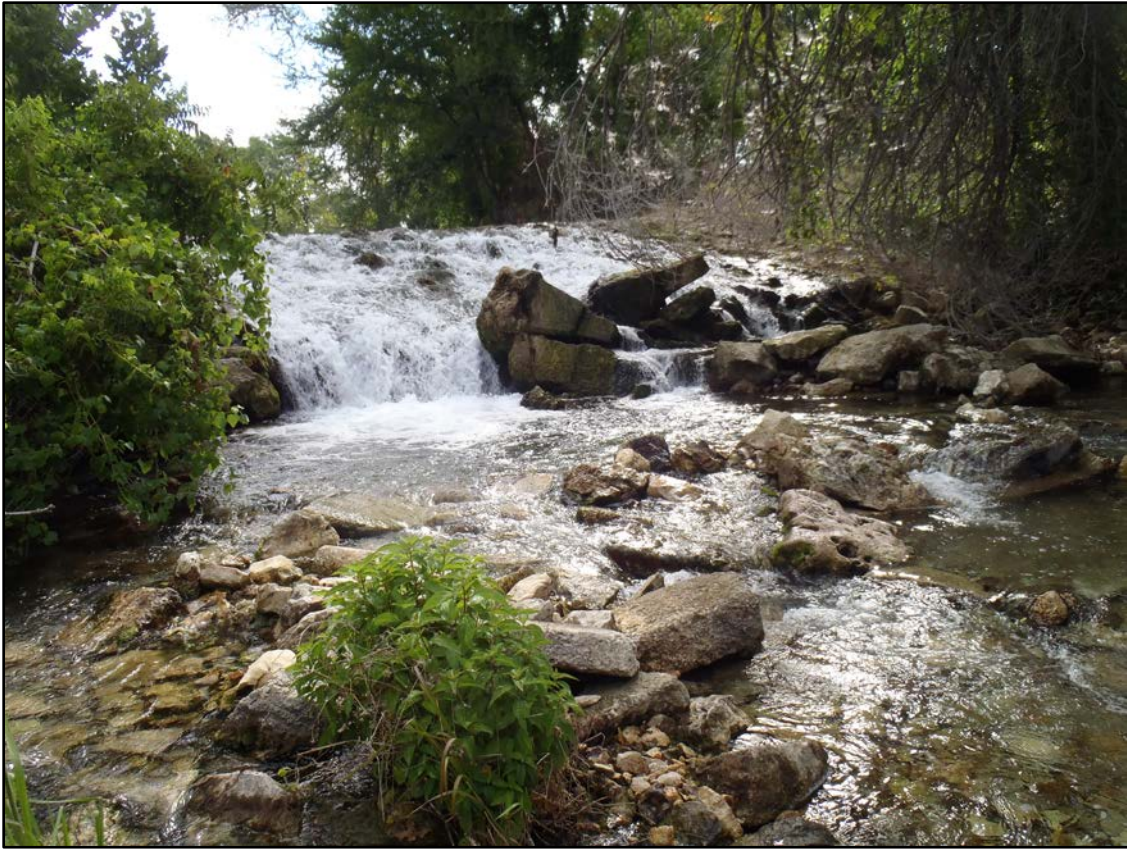
Figure 9: Spring Lake Dam Spillway on July 27, 2022.
