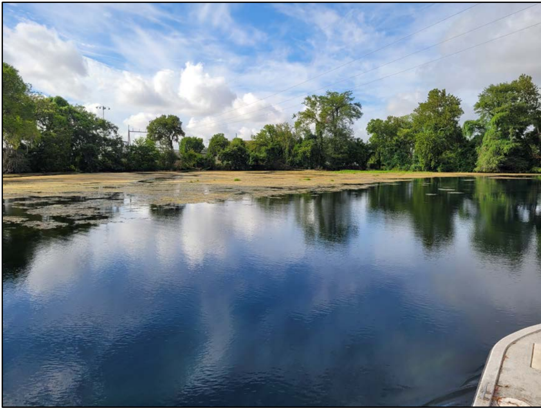
Figure 5: View of Spring Lake toward Spring Lake Dam spillway on July 27, 2022.
