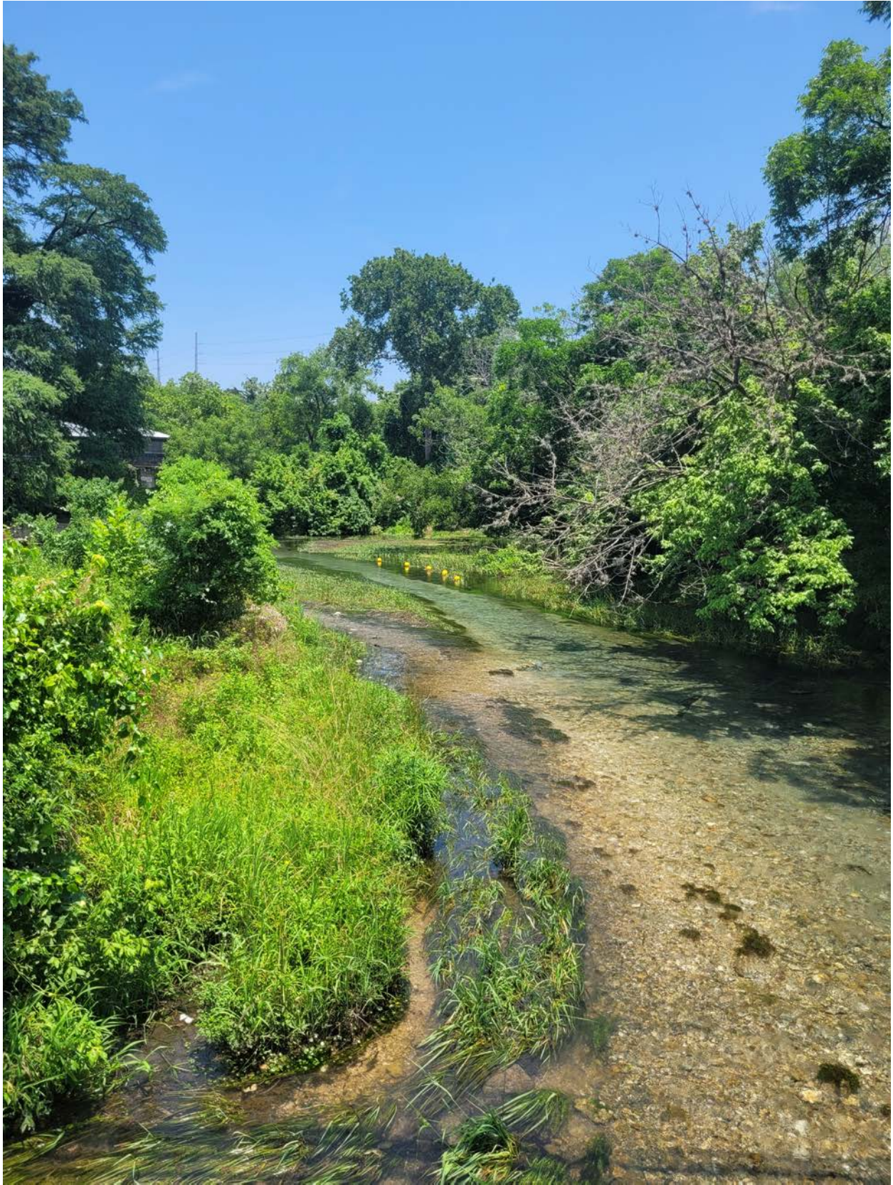
Figure 6: Spring Lake Dam looking upstream towards dam on June 22, 2023.
