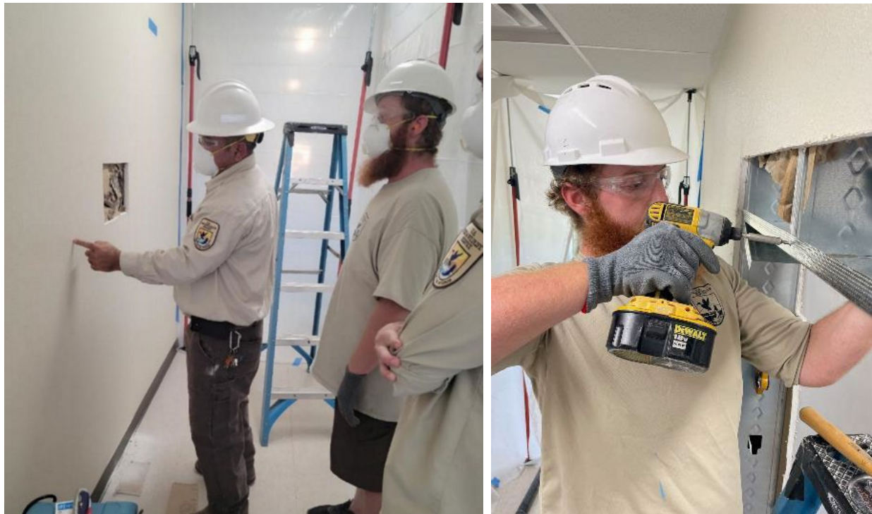
Figure 3. Left: Modifications to the EARP building begin. Juan Martinez (SMARC) instructing Braden West and Tommy Funk on how to properly create a doorway in a wall. Right: Braden West reinforcing the doorway after modifying a hallway.
