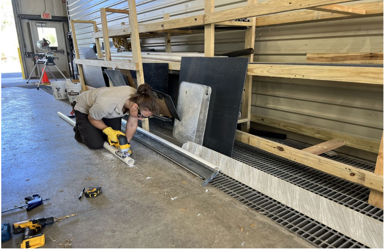
Figure 2. Heidi Meador cutting a drainage gutter for the new Hospital system in the Uvalde refugia.
