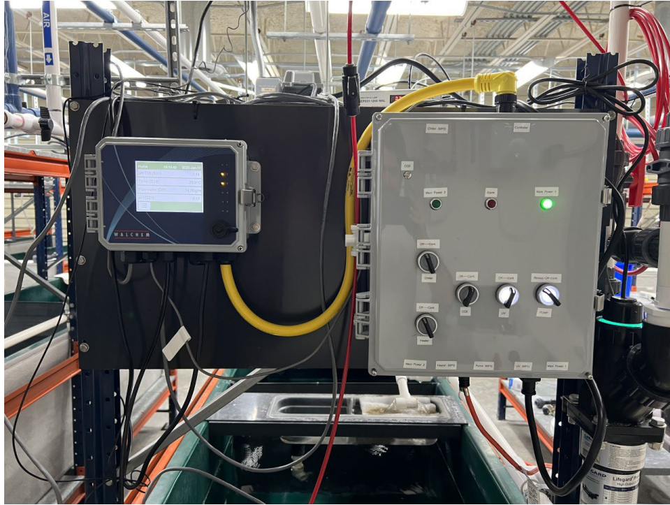
Figure 3. The electrical panel installed on a Walchem, Inc control/monitoring system on a tank in the UNFH refugia.
