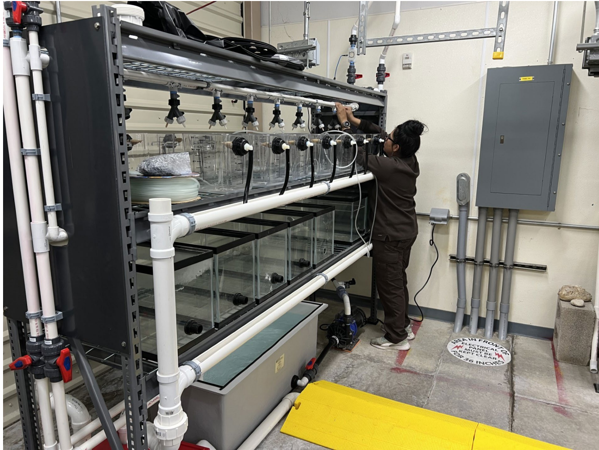
Figure 2. Dominique Alvear installing air and water lines for tanks on the new hospital tank rack.
