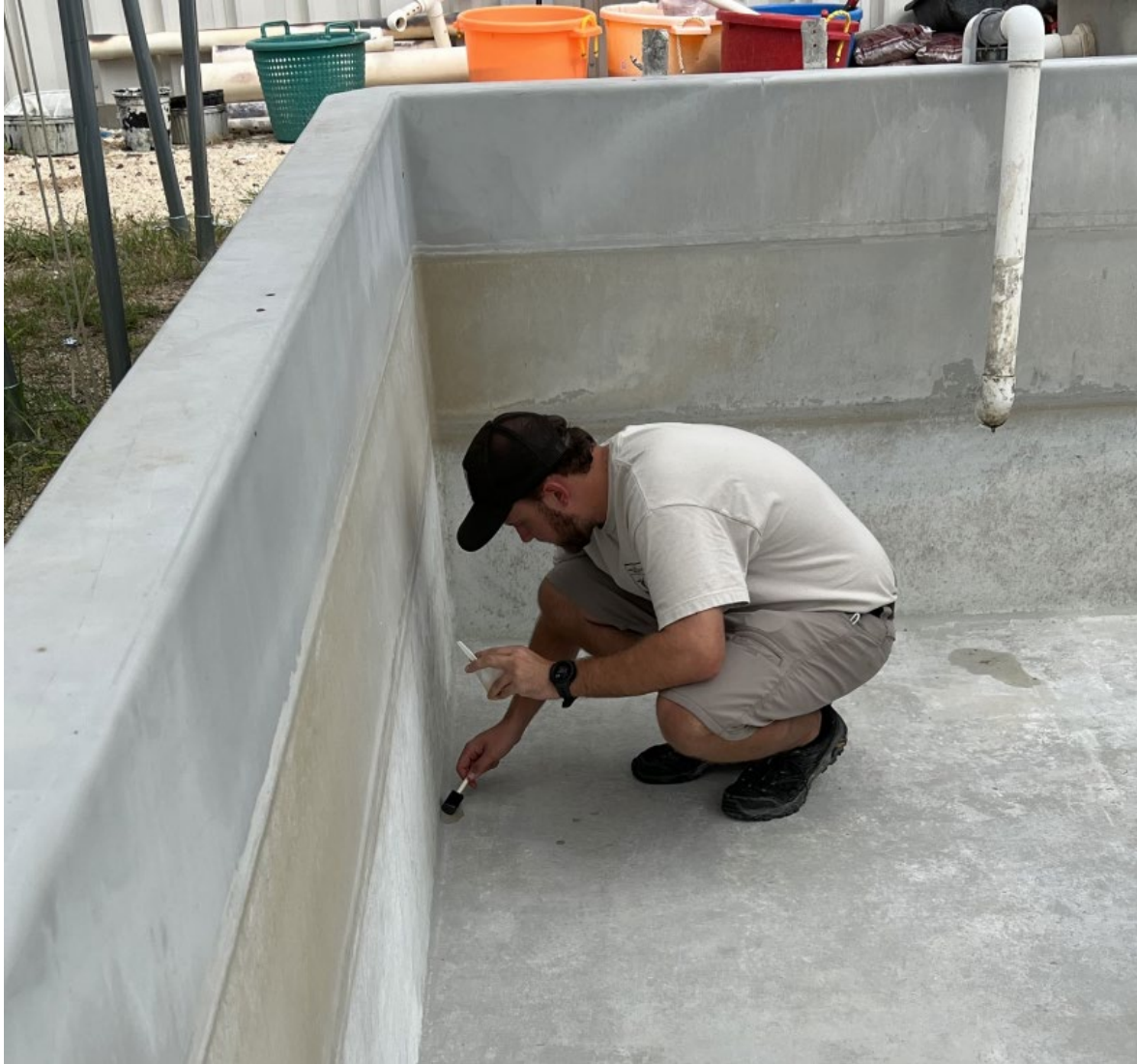
Figure 3. Jonathan Donahey repairing chips in a Texas wild rice holding tank.
