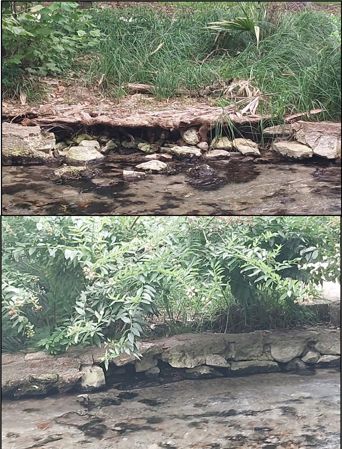
Figure 2. Low water levels have undermined several portions of the rock wall along Spring run 3. Some areas of the wall have completely caved in undermining vegetation roots. Areas like this are susceptible to collapse and further erosion.
