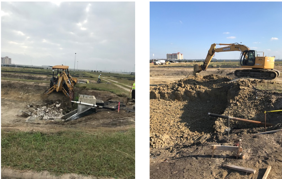
Figure 1. Nov. 03, 2017 Crews in the process of demolishing pond kettles and center levee
