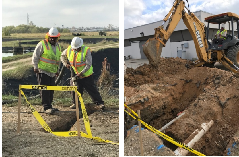
Figure 3. (Left) Utility crews using a hydro vacuum to locate existing lines. (Right) Once found, a backhoe is employed to expose area
