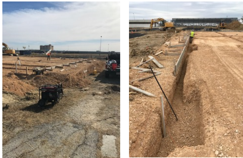
Figure 4. (Left) Crew placing forms. (Right) Excavation for footers
