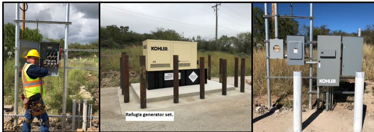
Figure 5 Refugia area electric supply and back-up generator at UNFH.
