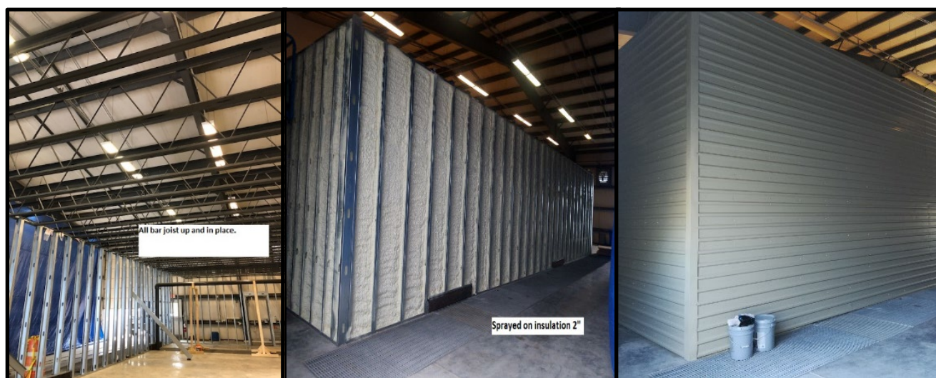
Figure 6 The progression of walls at UNFH for Refugia area: structure, insulation, and paneling.
