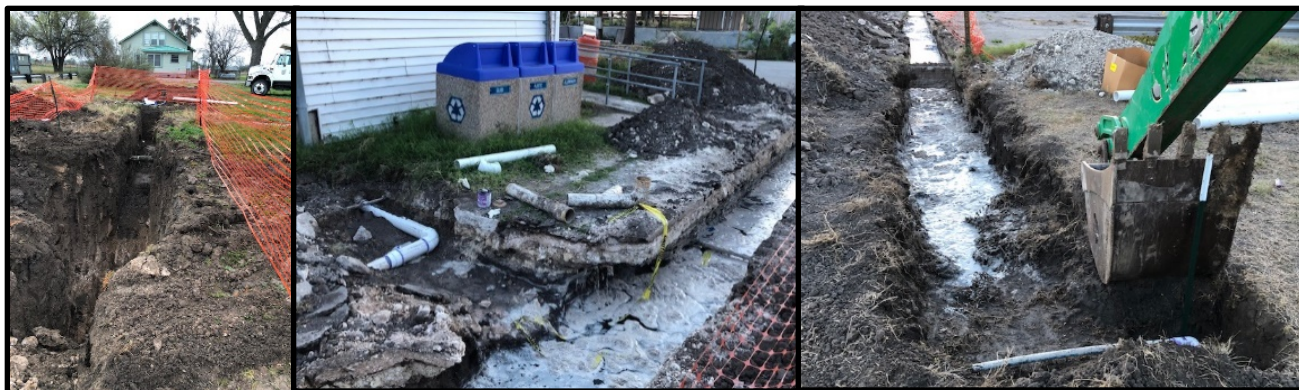
Figure 8 Trenching causing broken lines in need of immediate repairs at UNFH.
