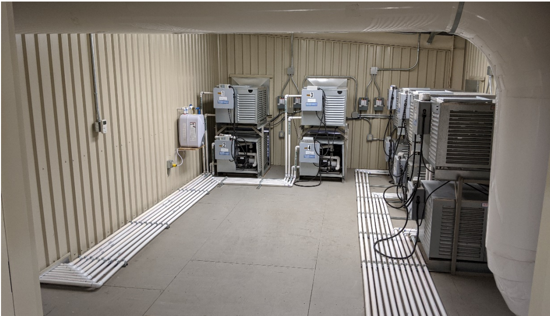
Figure 2. The mezzanine level of the quarantine space at the Uvalde National Fish Hatchery, where the heater/chiller units were installed. The top panel shows the room was open to the work area below. The bottom panel shows the room enclosed.
