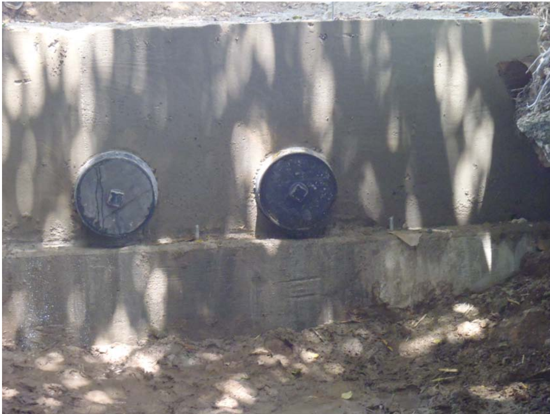
Figure 14: Sealed off old culverts in Landa Lake – photo of the Old Channel side.
