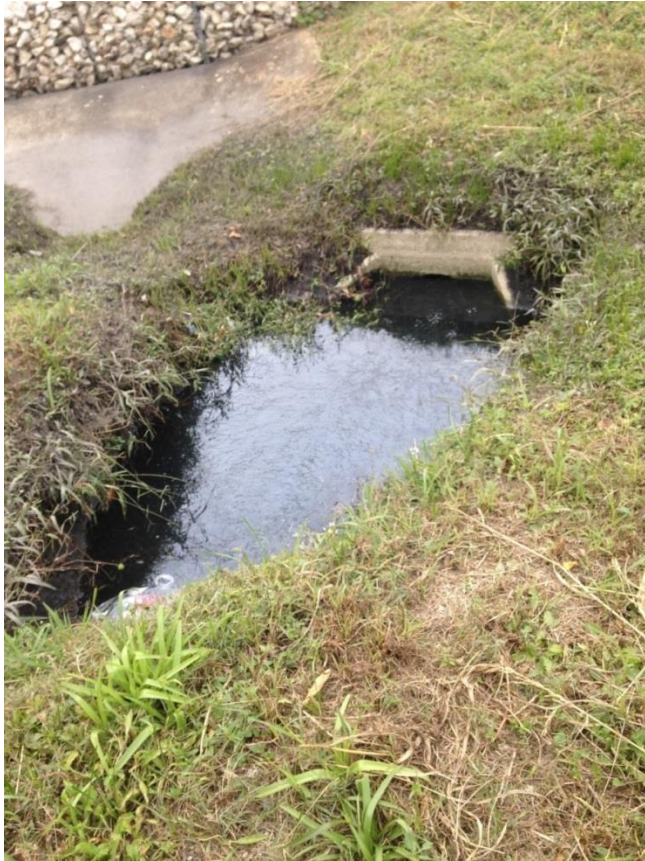
Figure 8-26 Photo of Erosion on Left Bank (Looking Upstream)
