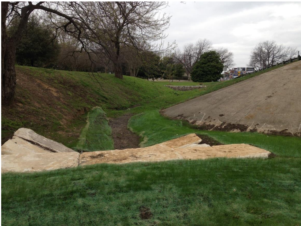
Figure 8-26 Photo of Erosion on Left Bank (Looking Upstream)
