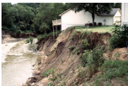
Figure 6-7 Creek Erosion Threatening Home
