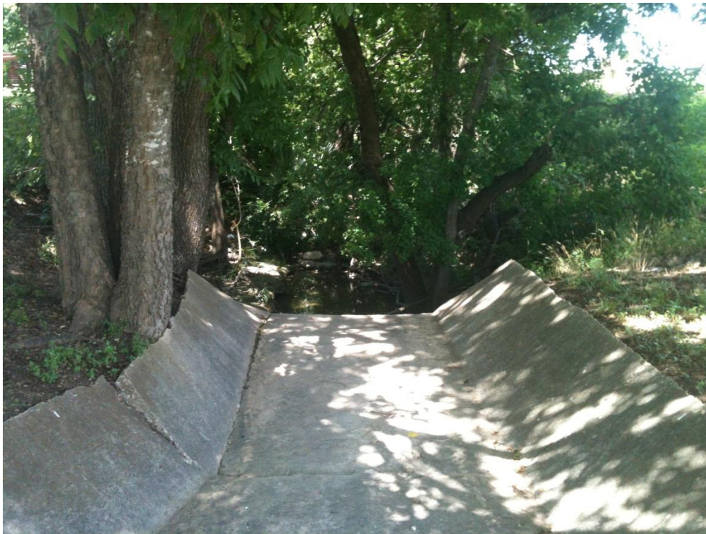
Figure 8-18 Photo of Existing Flume Looking Downstream
