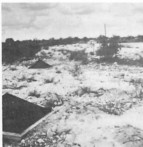
TRASH RACKS OVER DRILLED WELLS DRY FRIO RIVER
