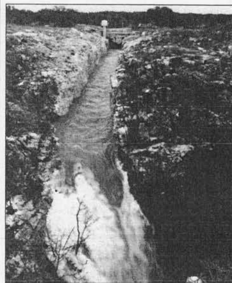
Diversion channel routing water from Seco Creek Dam to large sinkhole capturing excess floodwaters and allowing for rapid recharge to the Edwards Aquifer.
