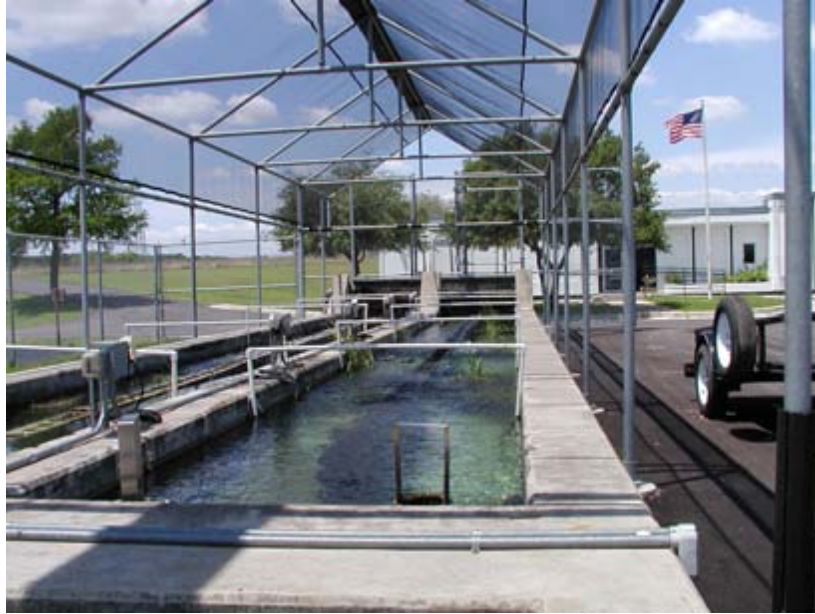
Figure 2-1. Concrete study raceways located at the National Fish Hatchery and Technology Center.
