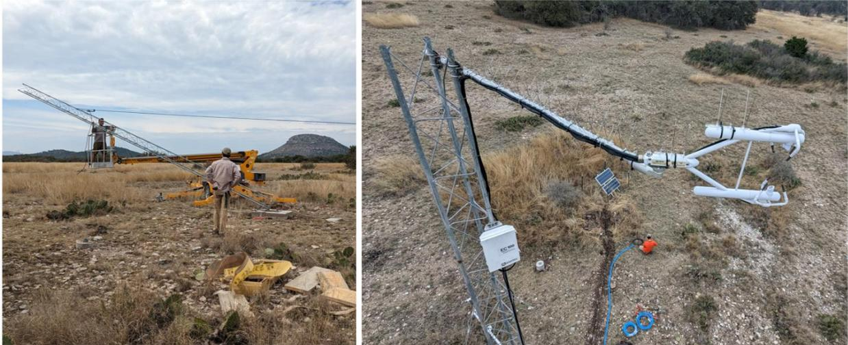
**Figure 2.5. Photographs of Nueces (US-EA6) Station Installation.** (left) Installation of the tower structure for the Nueces site by EAA personnel; (right) installation of ground-based sensors by EAA personnel in pit #1 within a grass patch by the station solar panel.
